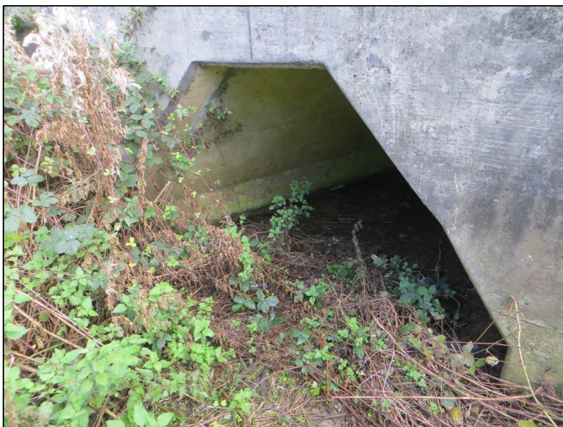
Figure 2.2 - Culvert Under M1 Roundabout
